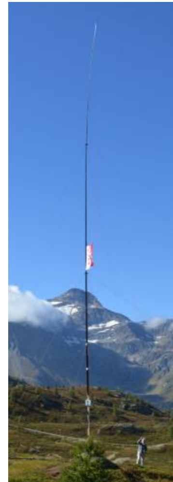
Full size 40 meter vertical antenna at HB9XBG
