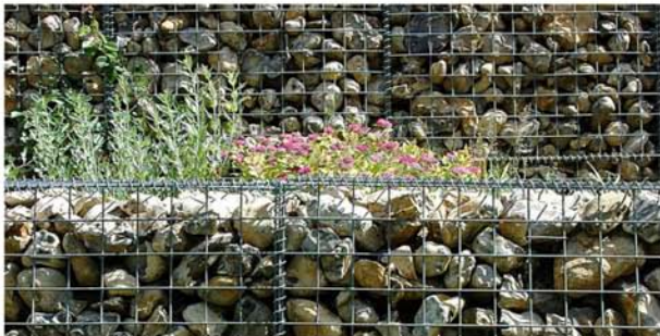
Gabion walls can be filled with many materials, including concrete, and planted upon or within. flickr.com/photos/21804434@N02/2797162704/
