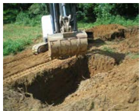
Figure 2: Photograph of trench excavation.
